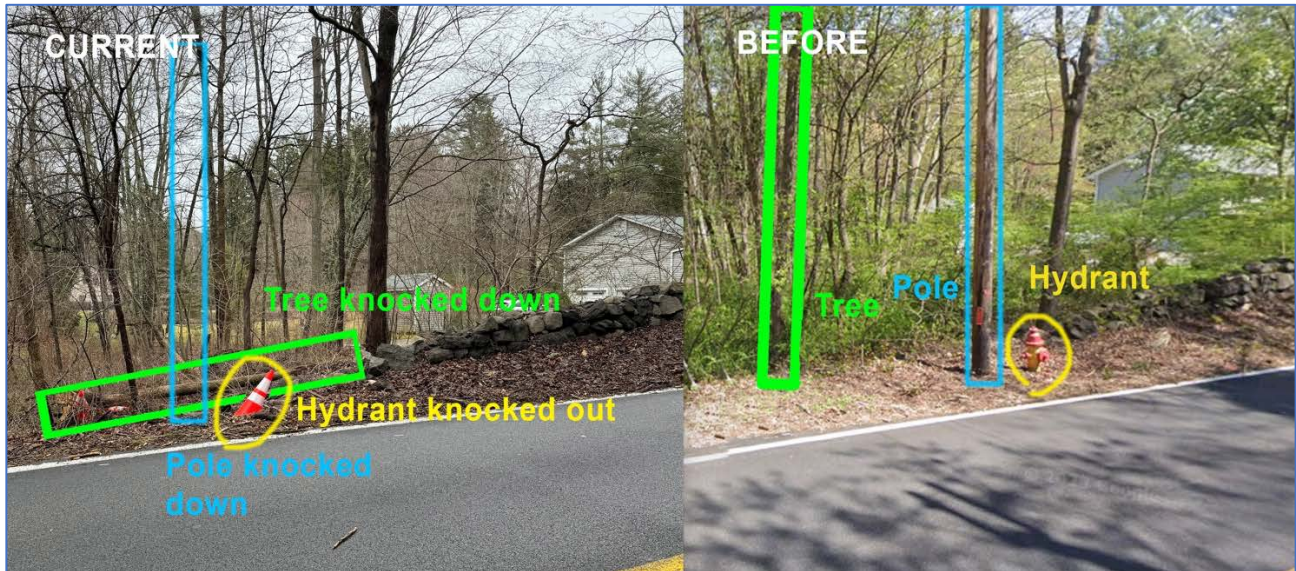
Photo 4 - Damage from 2nd accident on 12-28-24 - NOTE HYDRANT WAS FINALLY REPLACED ON 05-20-26 (1-1/2 years later)
